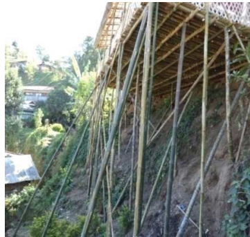
Plate 2. Bamboos used locally for construction of platforms and structures in hilly terrain.
