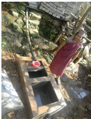
Kitchen Waste Water Soak Pit with Bio-Filter & Oil Trap Dymmiew & Massar Village, Pynursla C&RD Block, EKH
