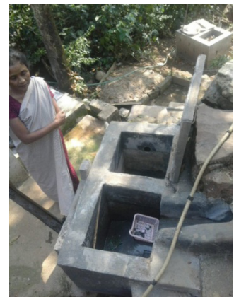
Kitchen Waste Water Soak Pit with Bio-Filter & Oil Trap Dymmiew & Massar Village, Pynursla C&RD Block, EKH
