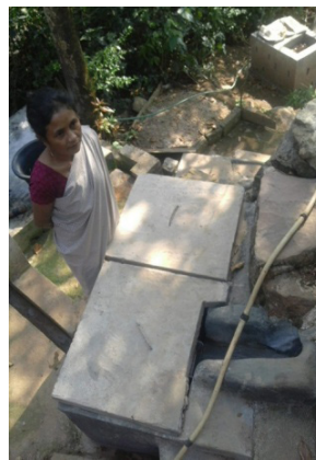
Kitchen Waste Water Soak Pit with Bio-Filter & Oil Trap Dymmiew & Massar Village, Pynursla C&RD Block, EKH
