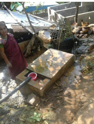
Kitchen Waste Water Soak Pit with Bio-Filter & Oil Trap Dymmiew & Massar Village, Pynursla C&RD Block, EKH
